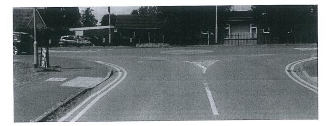
These crossing points are simply sections of footway and are dropped on either side of the road to allow users with mobility issues to cross the road more comfortably.
