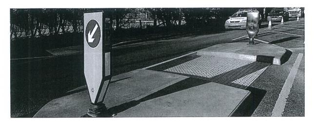
A pedestrian refuge island is a raised section of pavement between two lanes of traffic moving in opposite directions.
